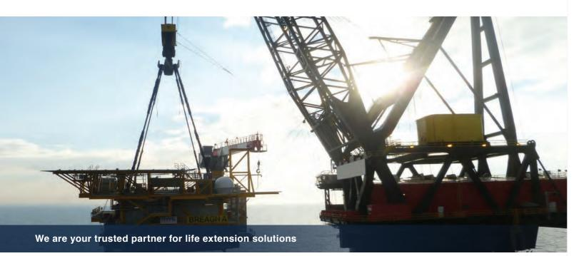
Repairs and strengthening for offshore structures and pipelines may be required for a number of reasons, the most common include fatigue, collision damage, and amendments to certification regulations. Planned changes, such as the installation of new process modules, may increase topside loads, and require further stiffening or bracing of the substructure.
